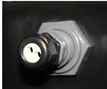
Double gland for level sensor & high level float
